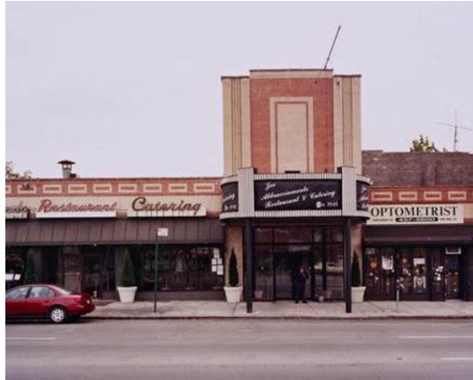
HISTORIC DRAKE THEATER, REGO PARK (DEMOLISHED)
