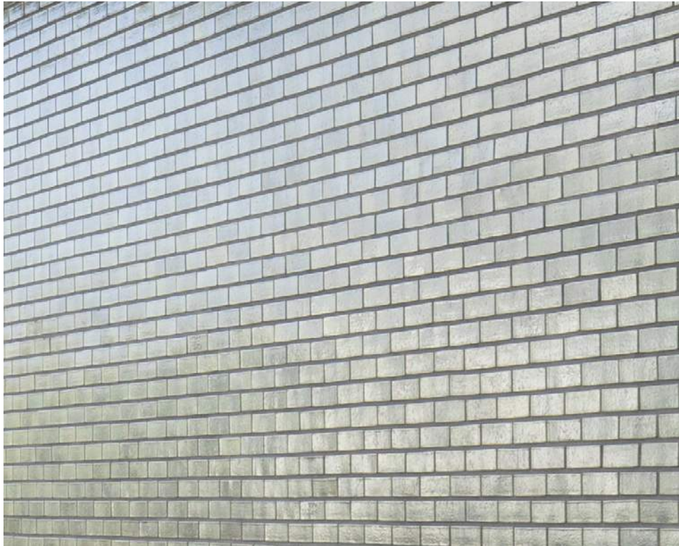
FACADE STUDY - MOTTLED FLAT BRICK
